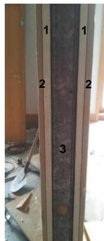
Lateral view of the system after having removed the vertical metallic framework
