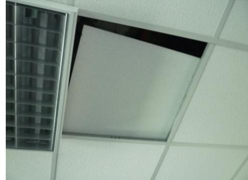
*Picture on the right: hanging ceiling made of mineral tiles. Source: French demolition company Occamat*
