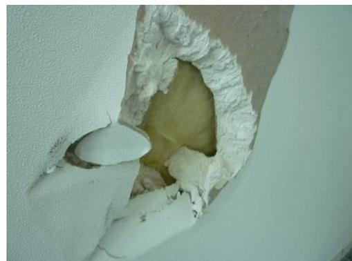
***Picture on the left: Double plasterboard system against a wall that has been drilled. Source: Recycling Assitance, Belgium***
